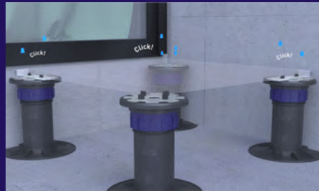
2. Remove the edge and corner spacers
